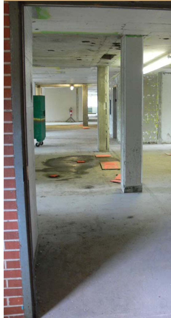
ABOVE LEFT: A snowman greets Catamounts coming back to Cullowhee. BELOW: Harrill Hall renovation in progress.
