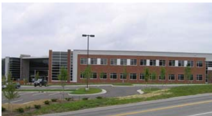
Multi-Tenant Facility, One of Several Virginia Tech Corporate Research Center Virginia Tech University
